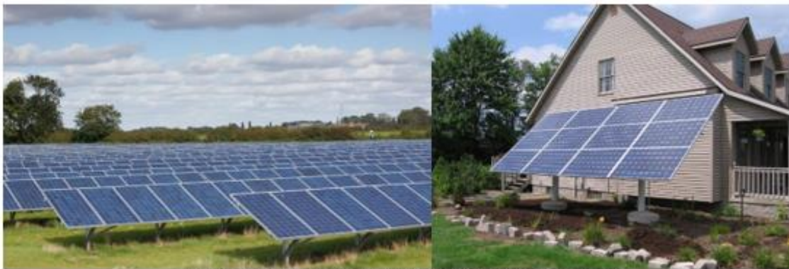
Figure 3: Examples of Ground-Mounted Solar Panel Installations
