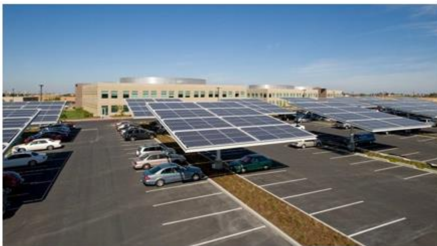
Figure 1: Example of a Dual Use Solar Panel Installations
